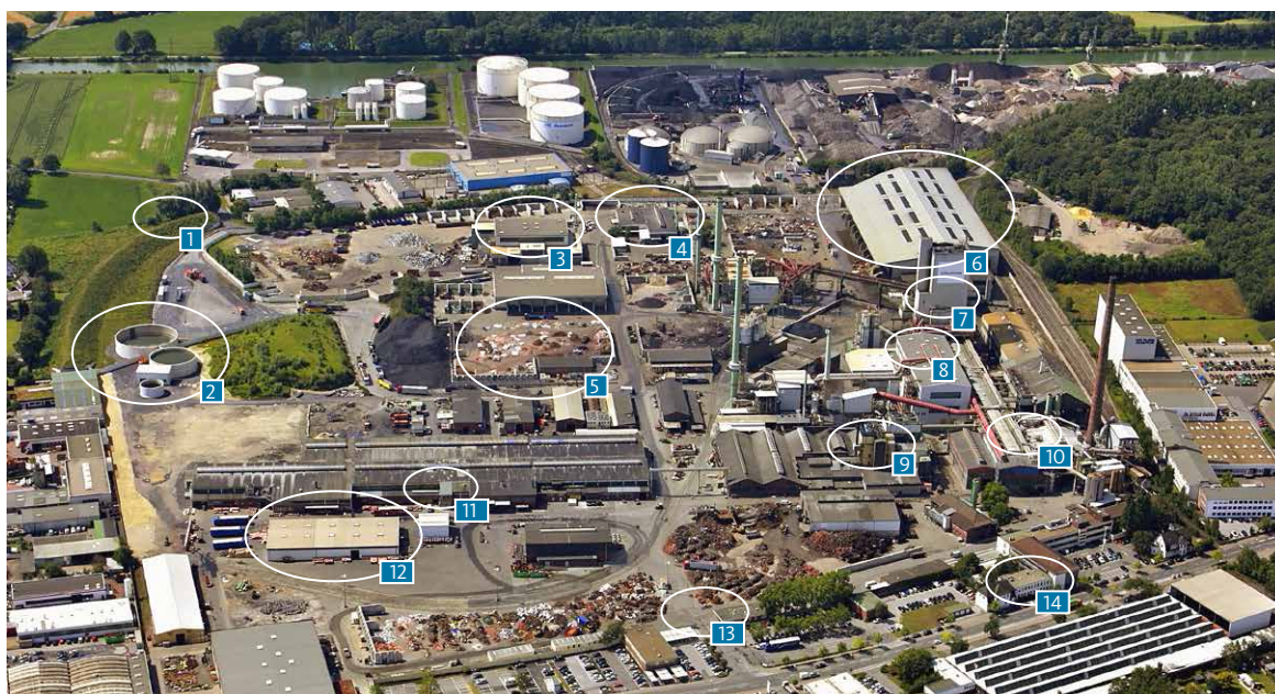
Fig. 3.1: Overview of Lünen site facilities
