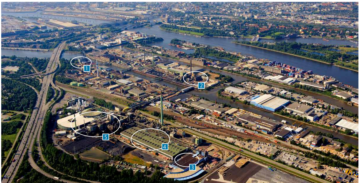
1 Continuous casting plant 2 Secondary copper smelter/precious metals 3 Rod plant 4 Tankhouse 5 Primary smelter (RWO)
