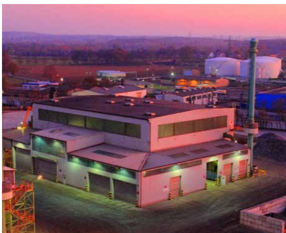
Aerial photo of the material preparation, crushing, and separation plant (MV-ZS facility) in Lünen
