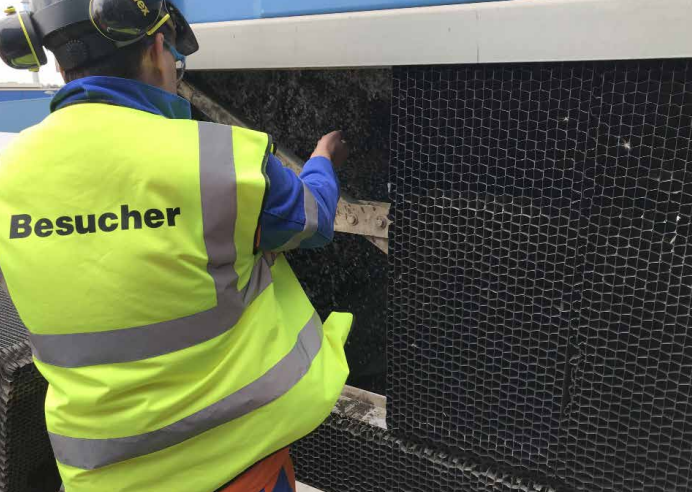
Expert inspection of the evaporation coolers
