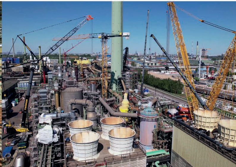
Snapshot during the shutdown at the Hamburg site.
