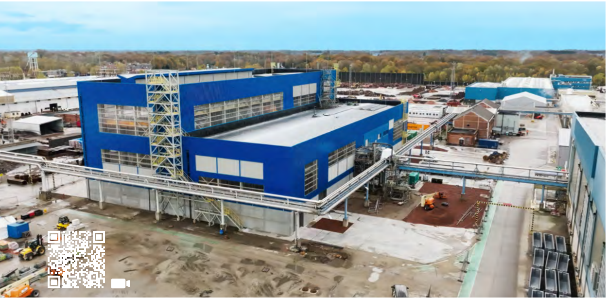
The new plant under construction in early November 2024.
